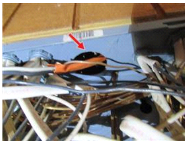
Missing panel bushings at added wiring in main panel area.
